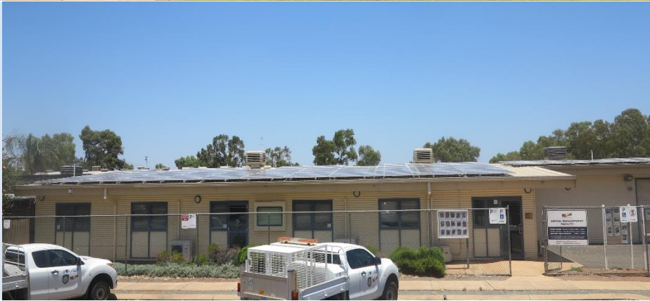
Kalgoorlie Animal Management Facility solar PV installation
