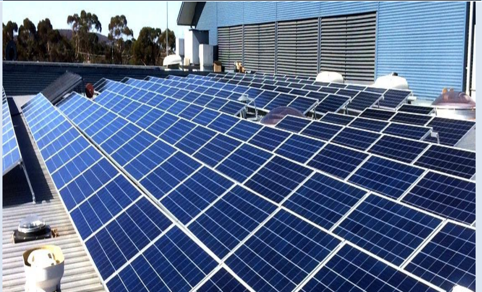
Shire of Coolgardie – Kambalda Recreation Centre
